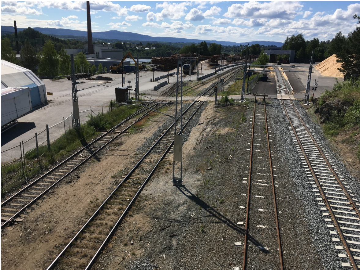
Fig. 4: South view from walkway overpass
